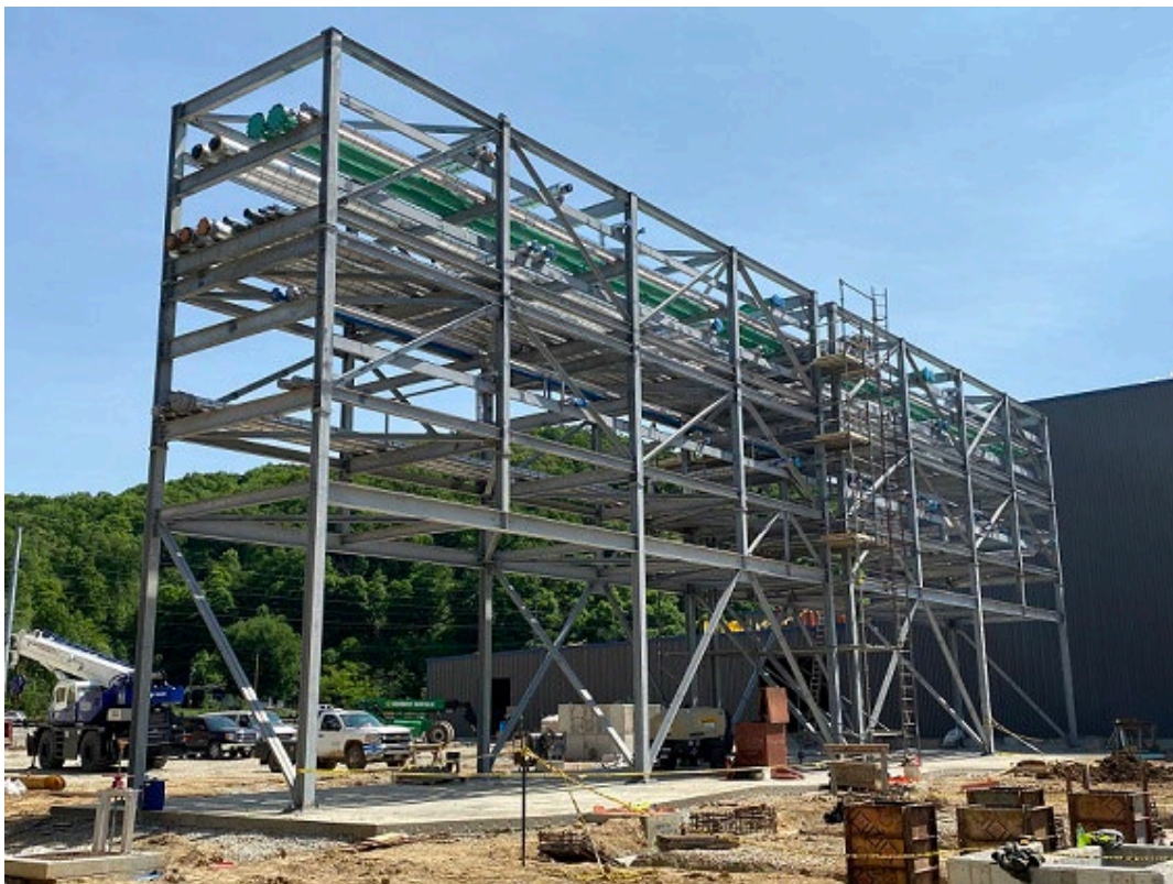
Figure 2: First Prefabricated Pipe Rack Modules at Building 610
