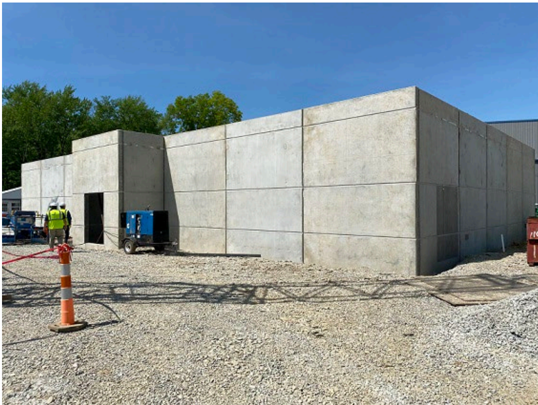
Figure 6: Erected Tilt-up Wall Panels of Building 620
