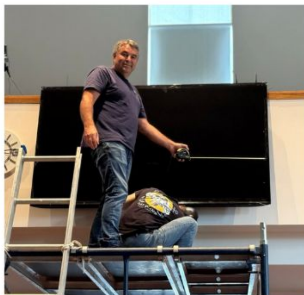
The new monitor in place. Randy holding the tape measure and Brian anchoring the monitor in place.
