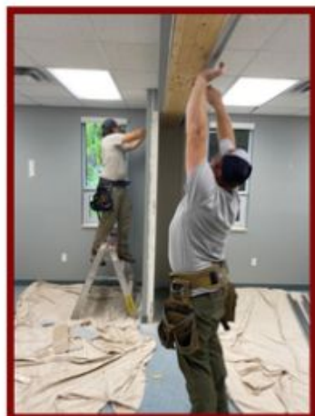
HERE YOU CAN SEE SOME OF THE WORK IN PROGRESS.
