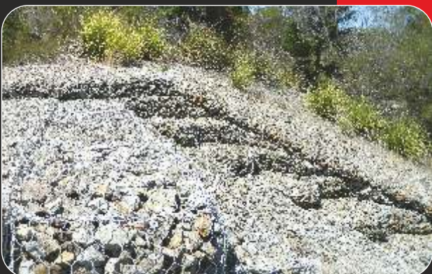
GABION AND ROCK MATTRESS INSTALLATIONS
