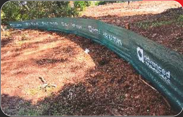
SEDIMENT CONTROL FENCING
