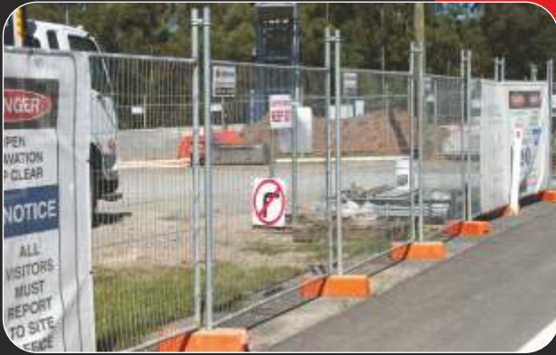
TEMPORARY MESH FENCING
