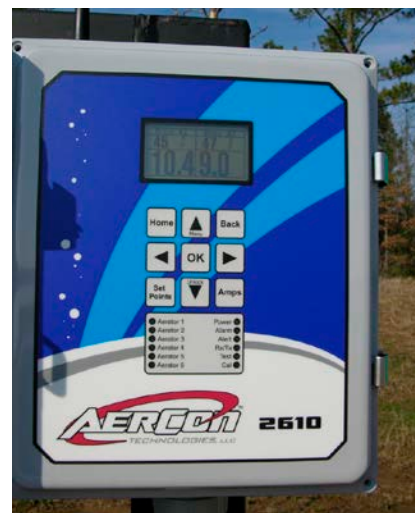
Figure 11 Control box for dissolved oxygen meters 1
