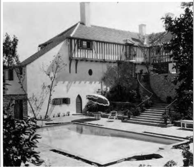
An exterior view of the rear elevation of the home of actor Frederic March and Florence Elderidge, and lately Jennifer Aniston and Brad Pitt with view of the swimming pool. Some experts speculate if there may have been drainage problems associated with the swimming pool.
