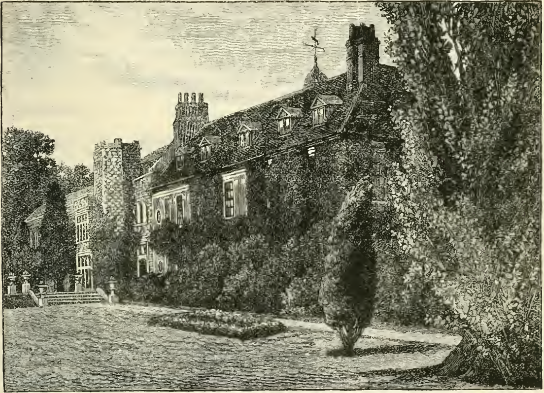
HALL PLACE, BEXLEY.
