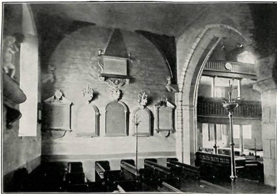
SOUTH TRANSEPT: OLD BECKENHAM CHURCH.
