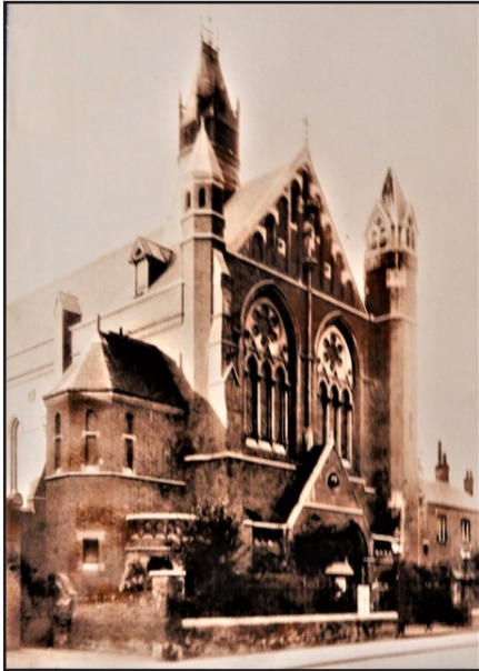
Bromley Congregational Church Widmore Road 1881-1940
