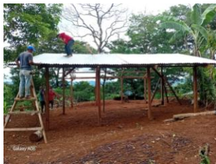
(New church building under construction)
