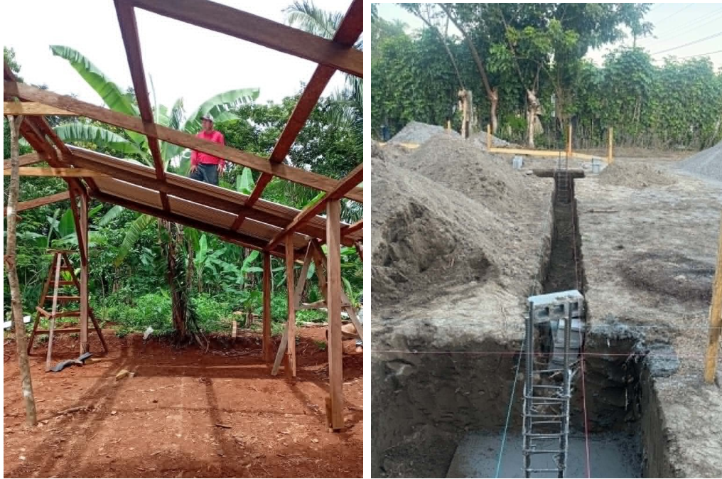
(Church construction continues in Panama)
