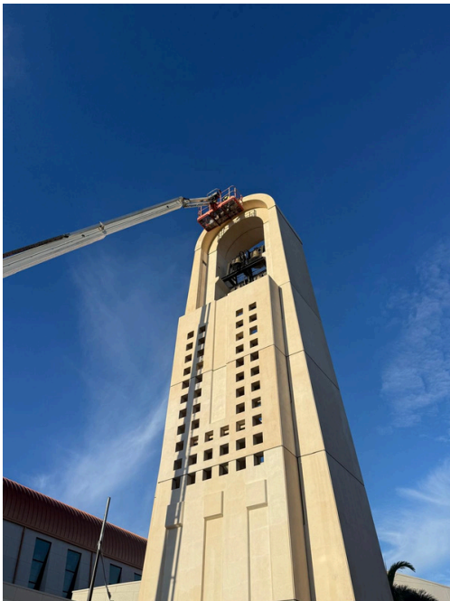
Filling in the gaps in the bell tower.
