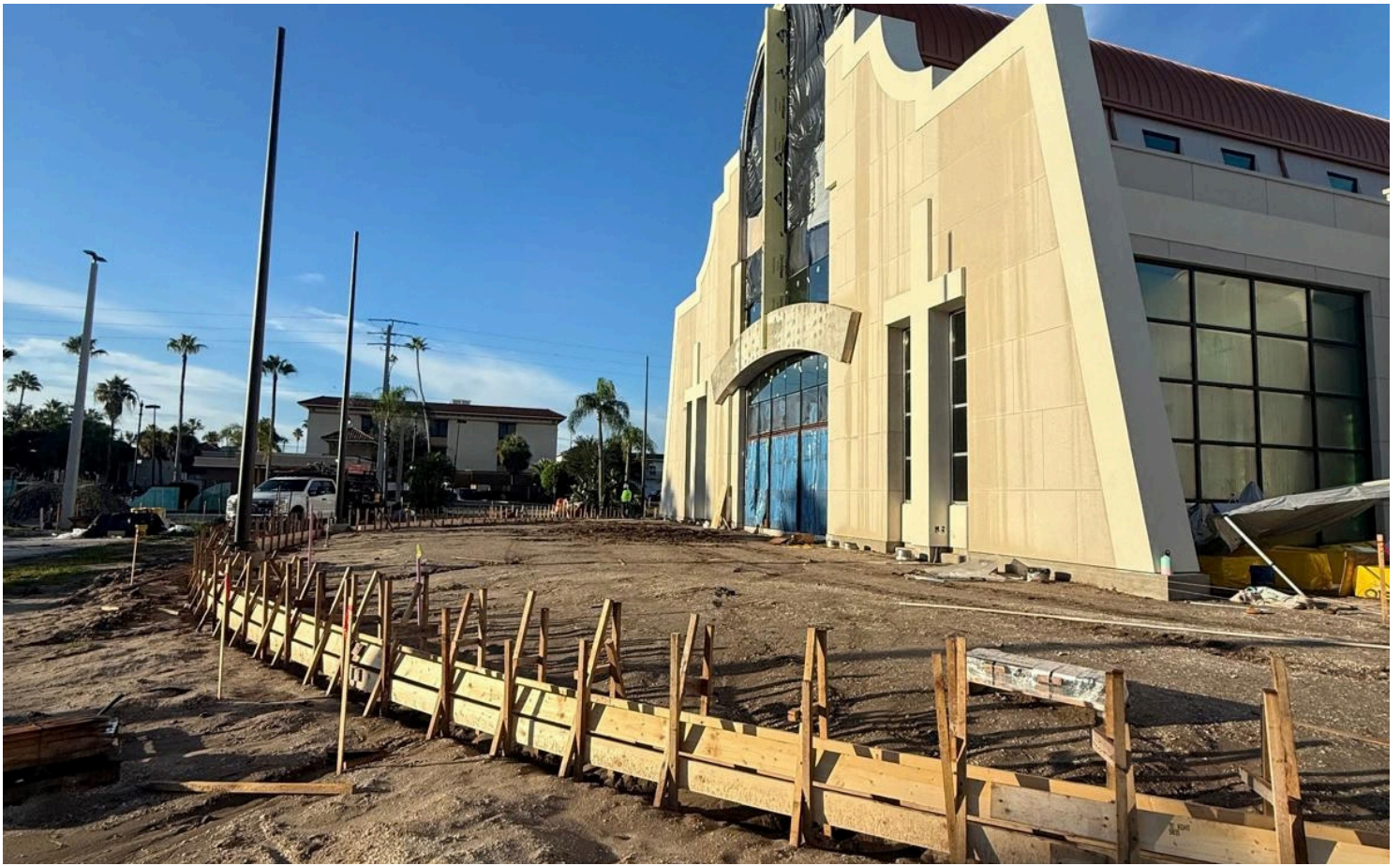
The formed foundation where the travertine patio will be laid.
