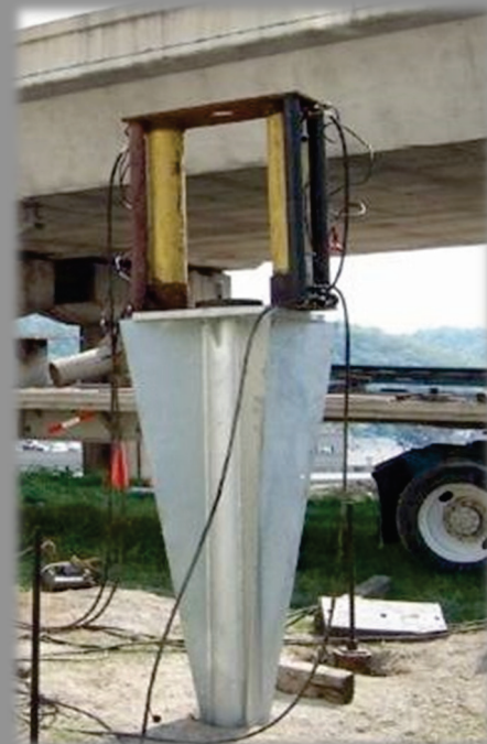
Galvanized foundation for a 120-foot tall road lighting tower in Charleston, West Virginia.
