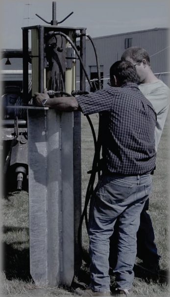
Moment foundation installed in under 30 minutes and ready for immediate construction. Wind turbine installation in Jackson, Michigan.
