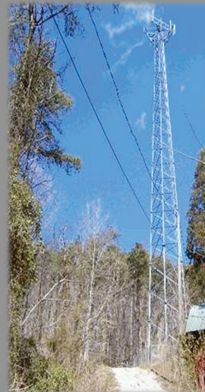
Structural Foundations installation for a cellular phone signal tower. Located atop Pea Ridge in the Appalachian Mountains, near Charleston, West Virginia.
