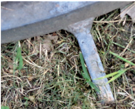
No corrosion or rust on the foundation top plate exposed to the elements since 1994 at Marietta College.
