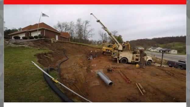
Hydraulically-installed steel foundations are emerging as an economical substitute for H-piles and other deep foundation systems in the construction of commercial and industrial buildings, with *total* installed costs typically 25% to 50% less than deep foundations and significant time savings.
