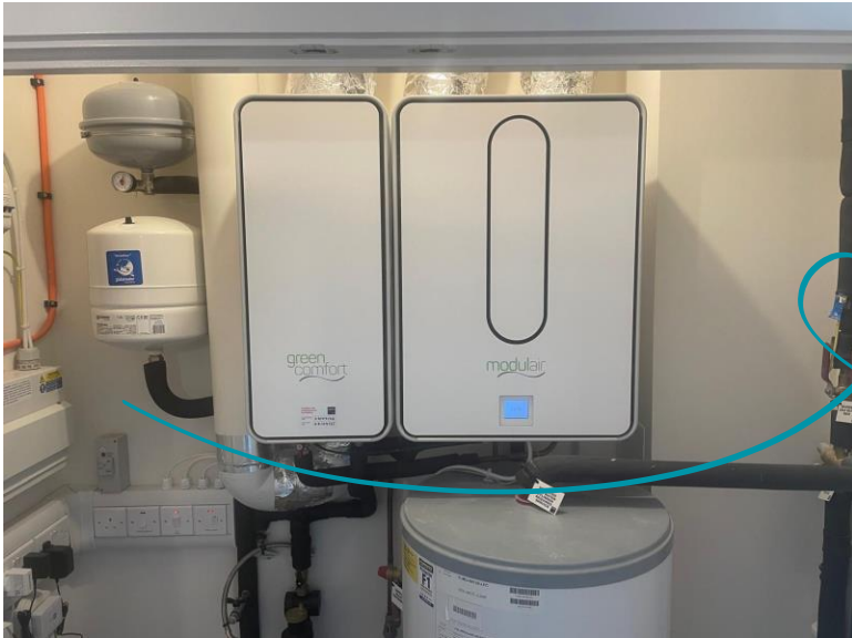
Church End Project – EAHP
