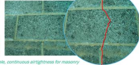
Parge coat = simple, continuous airtightness for masonry
