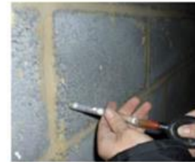
Parge coat = simple, continuous airtightness for masonry
