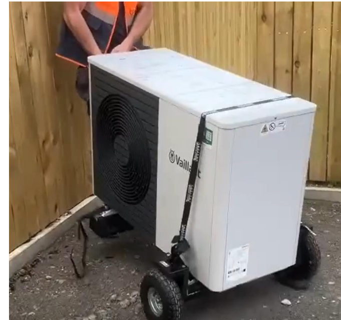
Heat Pump Mover
