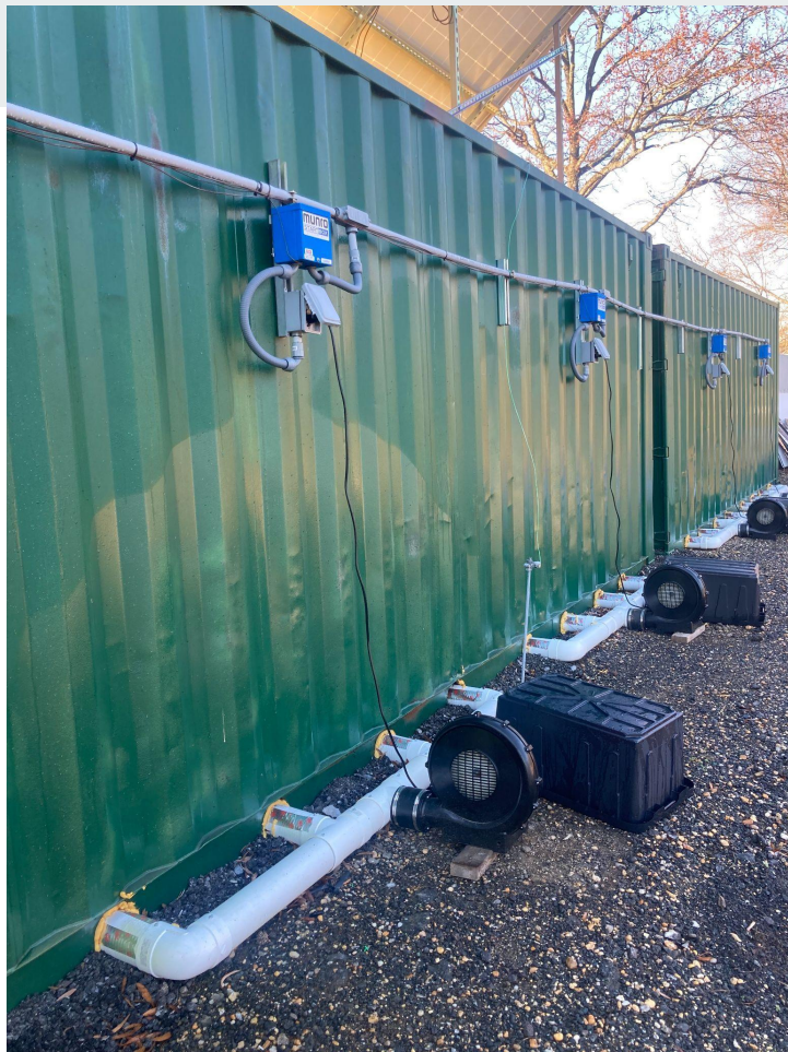
Piles are aerated at regular intervals by solar powered blowers
