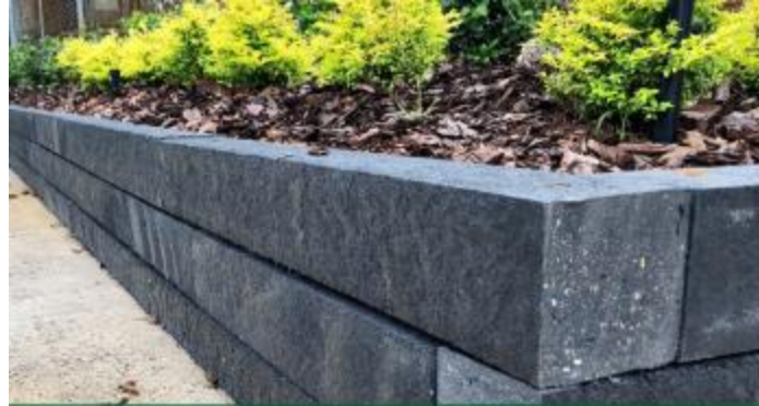
Raised Flower Bed & Retaining Wall
