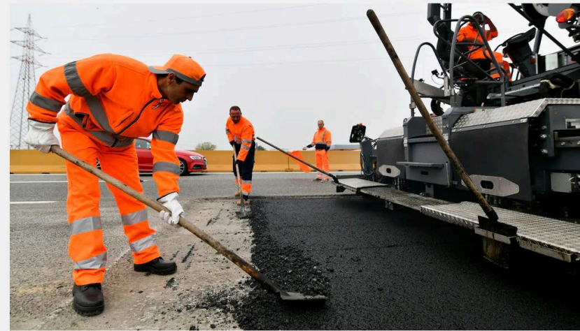
Workers lay down asphalt infused with plastic waste on a roadway in Turin, Italy. Stefano Guidi / Getty Images
