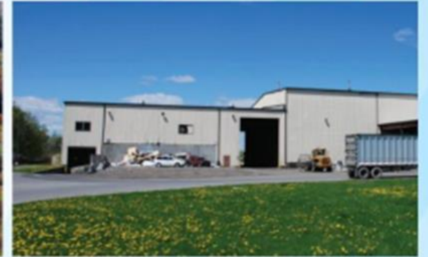
Three Solid Waste Transfer Stations
