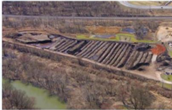
Green Waste Composting Facility
