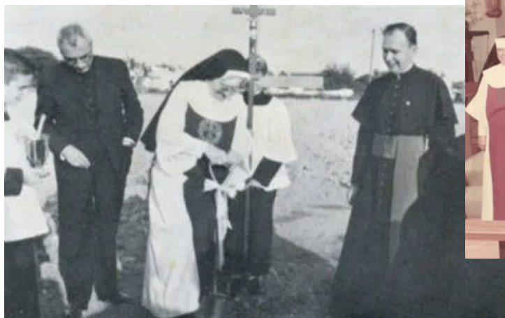
School Ground Breaking
