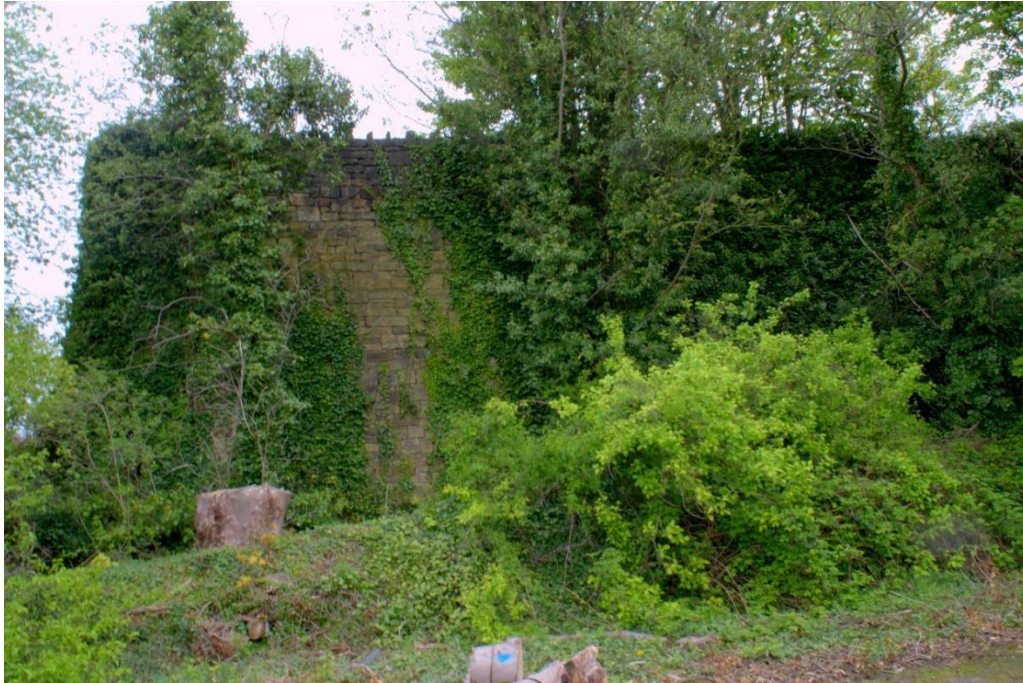
Figure 5 Revetment Wall at E end of site, Llangollen Rd to left.
