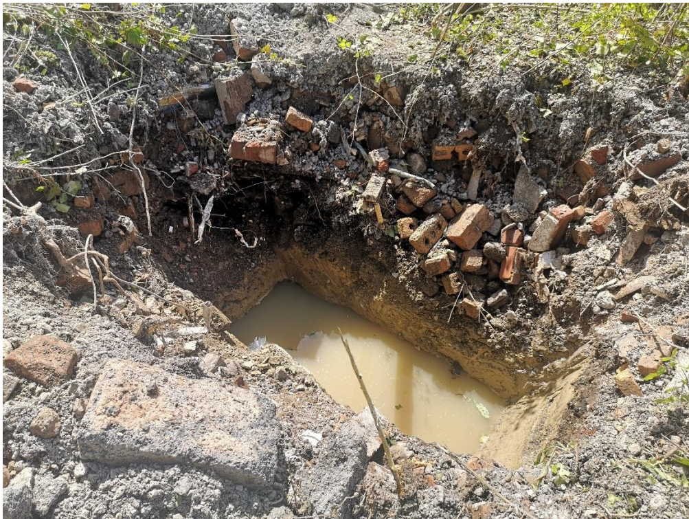
Figure 14 Engineer’s test pit with demolition debris and yellow clay subsoil. (photo D. Bailey).
