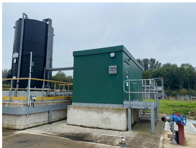
Fig. 15 Phosphorus removal unit at Otley STW (Photo, Yorkshire Water)
