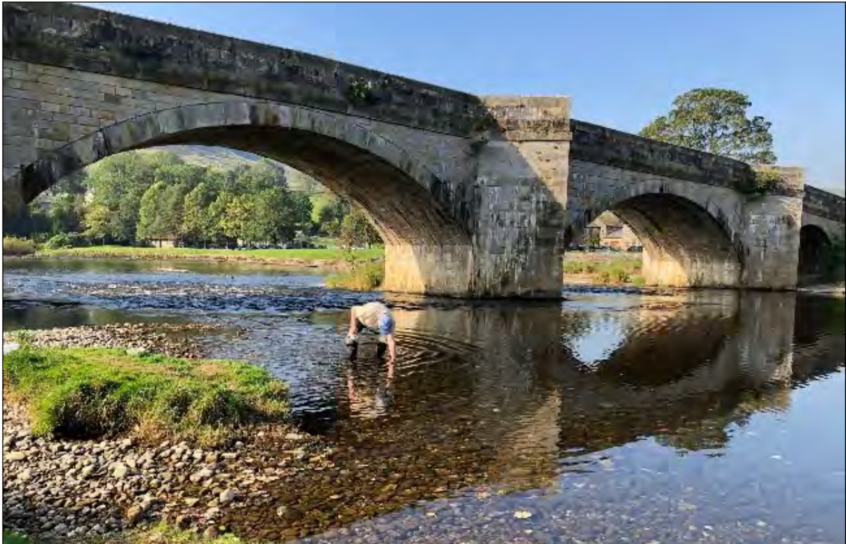
Zone 2: Burnsall Bridge
