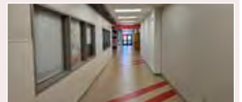
✓ BELTON HIGH SCHOOL INTERIOR FINISHES Completed August 2024
