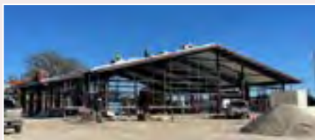
⌚ CONSTRUCTION OF NEW DELTA PROGRAM FACILITY Anticipated completion in early 2025
