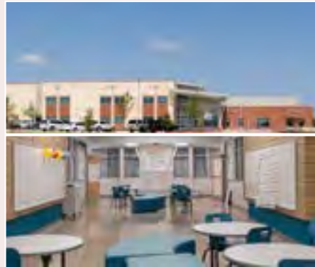
✓ HUBBARD BRANCH ELEMENTARY New K-5 elementary school Opened August 2024
