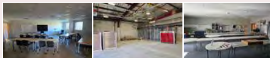
✓ BELTON HIGH SCHOOL CTE RENOVATIONS/UPGRADES Renovation project to provide new construction technology, agriculture, and vet tech classrooms Classroom instructional spaces reached substantial completion in September 2024, new shop spaces supporting construction technology completed November 2024.
