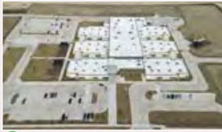
✓ JAMES L. BURRELL ELEMENTARY New K-5 elementary school Opened January 2024
