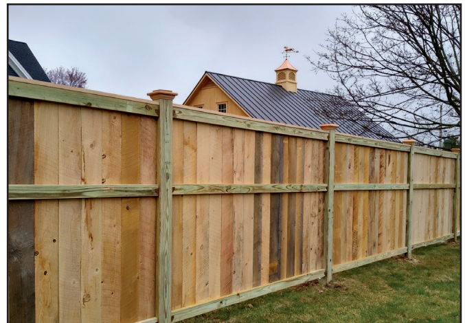
6FT TALL HEMLOCK PRIVACY FENCE IN CAP AND TRIM (BACKSIDE)
