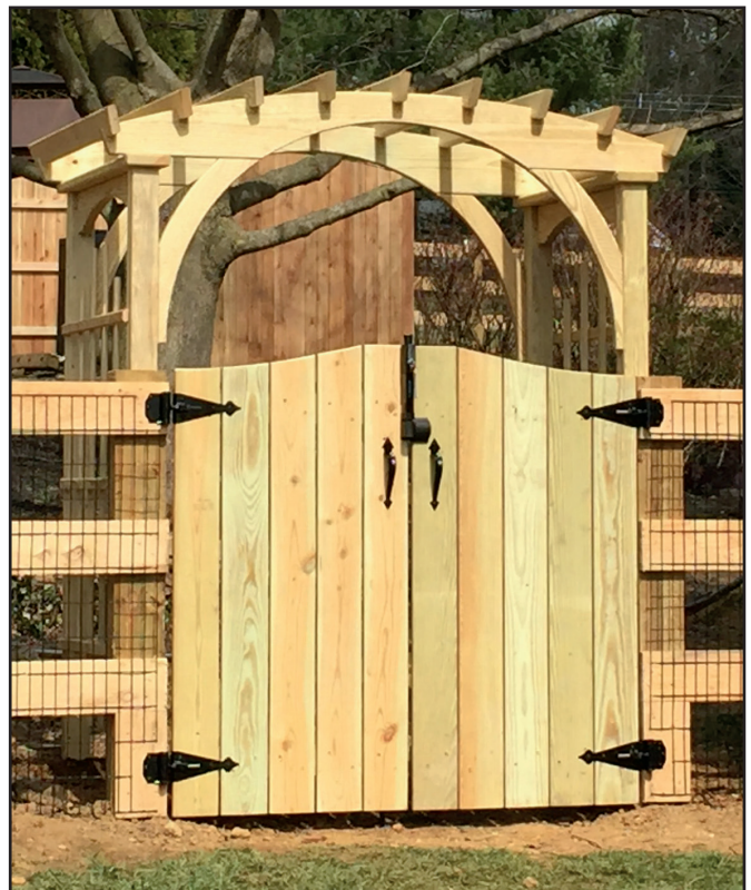
CUSTOM ARBOR WITH PRESSURE TREATED PRIVACY GATE
