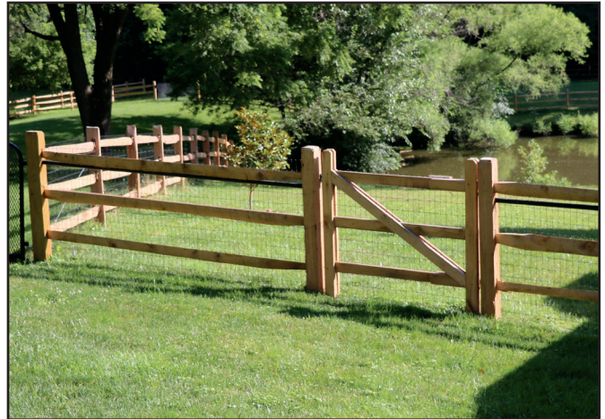
3 RAIL SPLIT RAIL FENCE WITH 2X4 BLACK WOVEN WIRE
