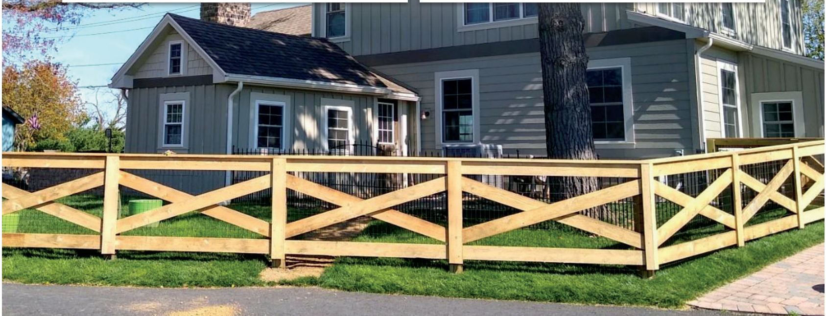
4-BOARD NAIL ON CROSS BUCK FENCE WITH FACEBOARD AND DRINK RAIL PLUS 2X4 BLACK VINYL WIRE
