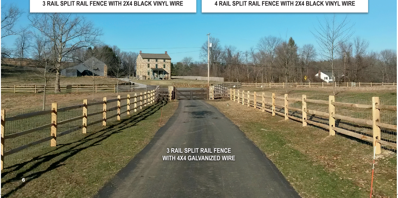
3 RAIL SPLIT RAIL FENCE WITH 2X4 BLACK VINYL WIRE
