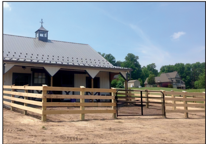
4 BOARD NAIL ON FENCE WITH CAP (4X6 POST WITH HEMLOCK BOARDS)
