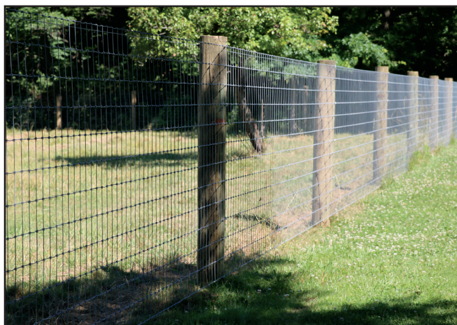
ROUND POST WITH 2X4 GALV WIRE MESH AND HI-TENSILE ELECTRIC
