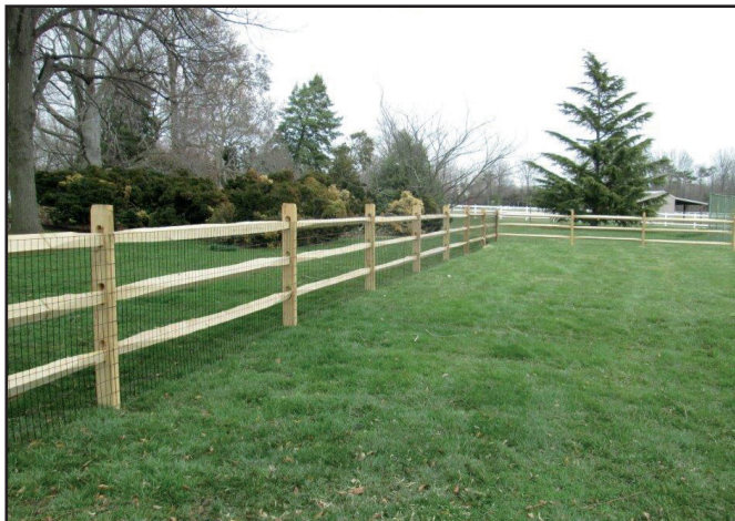
3 RAIL SPLIT RAIL FENCE WITH 2X4 BLACK VINYL WIRE
