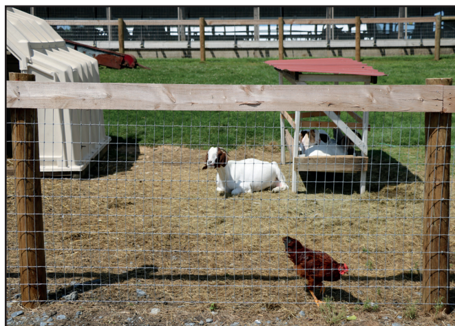
ROUND POST WITH 2X4 GALV WIRE MESH AND HEMLOCK BOARD
