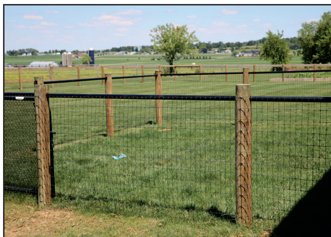
ROUND POST WITH 2X4 BLACK WIRE MESH AND CUSTOM BLACK PIPE
