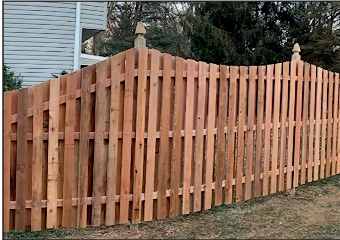
6FT TALL RED CEDAR SHADOWBOX FENCE IN CONCAVE DESIGN
