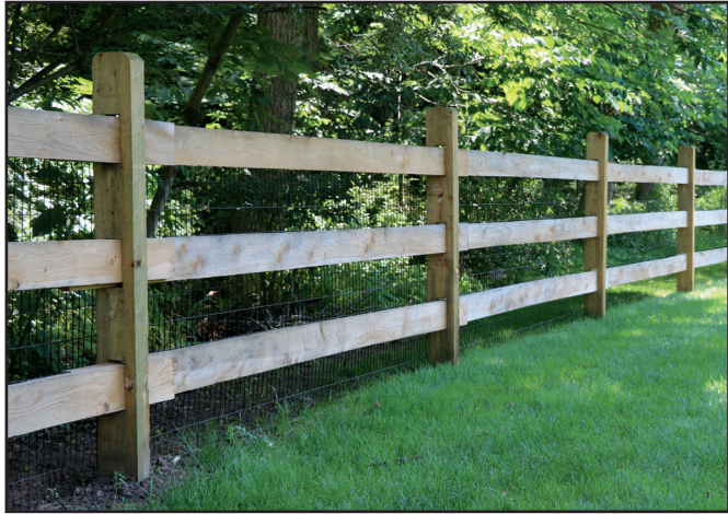
3 RAIL SLIP BOARD FENCE WITH 1.5X4 POOL CODE WIRE
