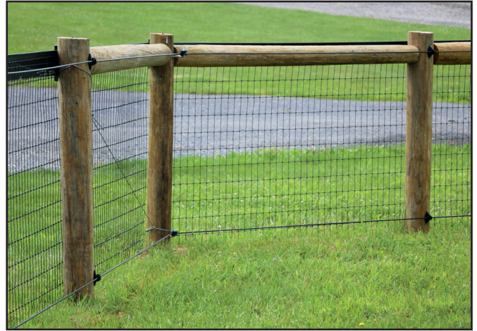
ROUND POST WITH 2X4 BLACK WOVEN WIRE AND BLACK FLEX RAIL PLUS 2 STRANDS OF BLACK COATED HI-TENSILE
