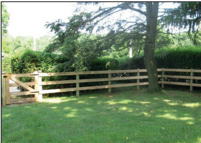
3 BOARD NAIL ON FENCE WITH 2X4 BLACK VINYL WIRE
