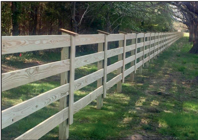
4 BOARD NAIL ON FENCE WITH FACEBOARD AND CAP (P.T. POST AND P.T. DECK BOARDS)
