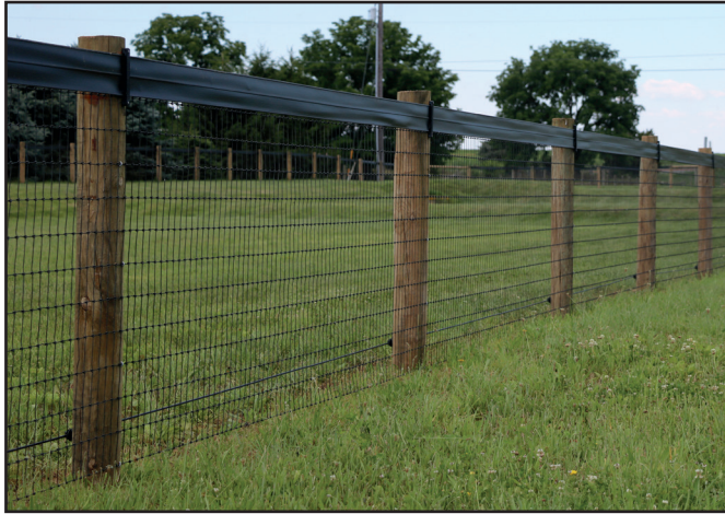
ROUND POST WITH 2X4 BLACK WIRE MESH AND BLACK FLEX RAIL
