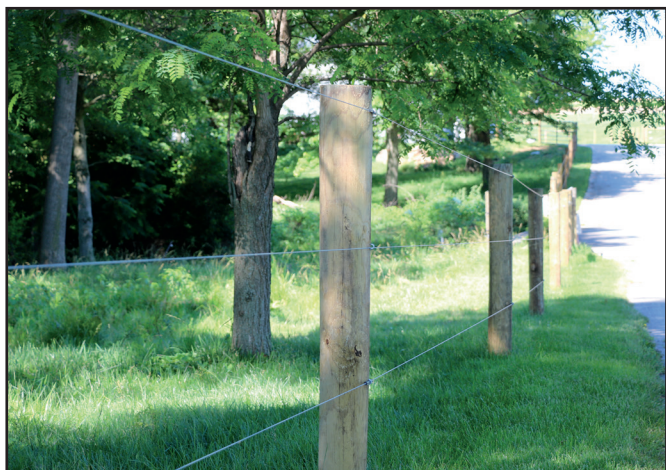
ROUND POST WITH 3 STRAND HI-TENSILE FENCE
