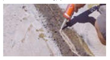
Flexural Cracking: These cracks are caused by engineered design structural faults and will readily sheer most membranes. In proper design, expansion joints stress relievers are inserted in the area where a flexural crack will develop (engineers can calculate this). In these circumstances, the application of UltraFlex FC is suitable.
