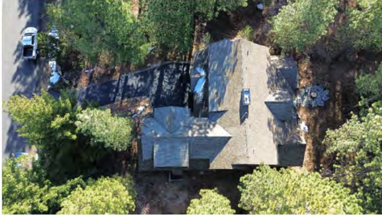
Roof Drone Overview
