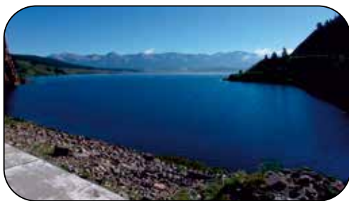
Taylor Park Reservoir August 2017
