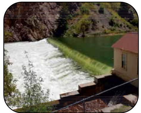
Uncompahgre Water Users' Gunnison Tunnel Diversion Dam June 2017
