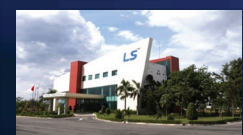
LSCV (HO Chin Minh) MV / LV Cable UTP, Optical Cable Overhead Cable
