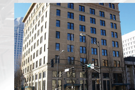
WINSTON SALEM APARTMENTS PMC Property residential building Winston Salem, North Carolina Ex-Way (UL) supply
