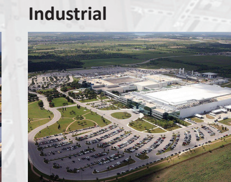
SAMSUNG T-PROJECT Electronics semi-conductor plant Taylor, Texas Ex-Way (UL) & DTS supply, installation
