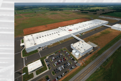
LG ELECTRONICS TN LG home appliance factory Clarksville, Tennessee Ex-Way (UL) supply
