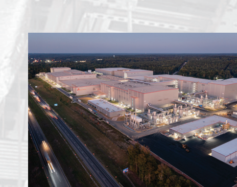
SK BATTERY AMERICA SK Innovation (Phase 1 & 2) Commerce, Georgia Ex-Way (UL) supply, installation
