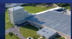
LSCUS (Tarboro) MV / LV Cable Control, Instrument Cable
