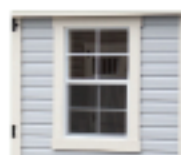
Painted New England Window Trim
