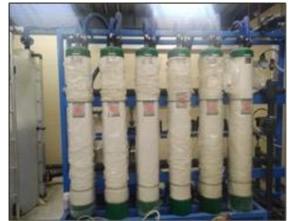
Ultrafiltration and reticulation system helps carry a production capacity of 155,000 litres of water per day
