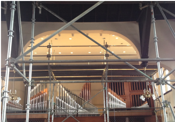
Construction workers build scaffolding to repair and replace broken lights before installing a new sound system on the ceiling.
