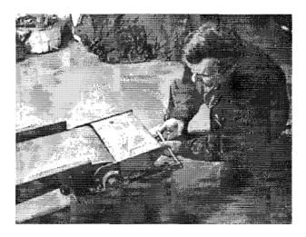
Step 5: Slacken off the Belt Tensioning Bolt
