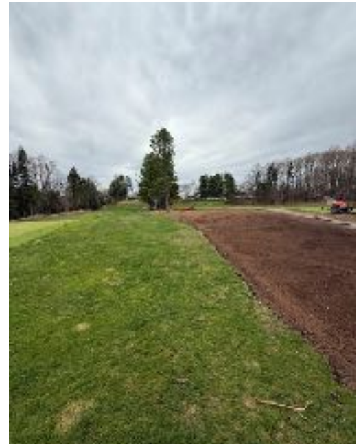
Site prep work on the left side of 12
