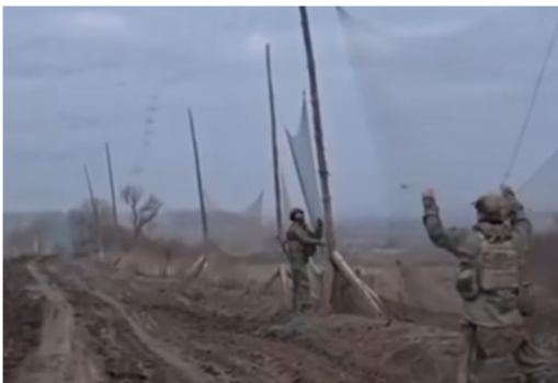
Russian soldiers erecting a 2km net tunnel over supply lines in Ukraine.
