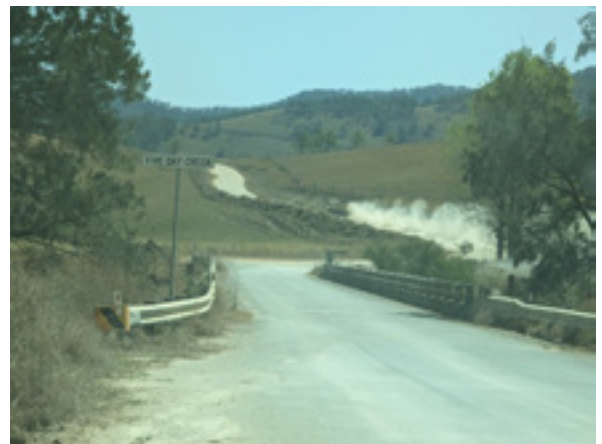
Plate 6.4 Kempsey Road – Dust Generation on Unsealed Roads
