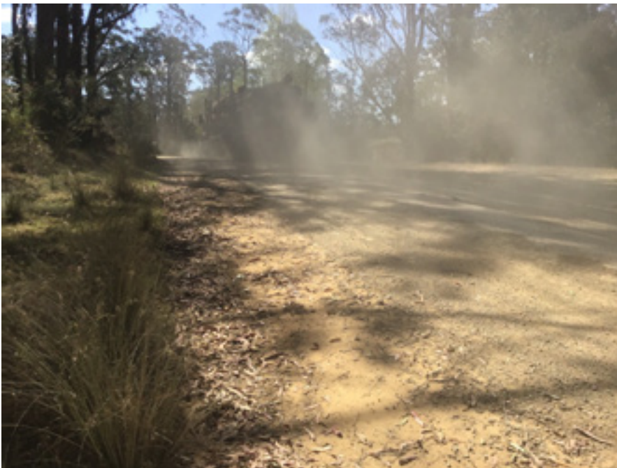
Plate 6.9 Dust generation on Kempsey Road unsealed sections
