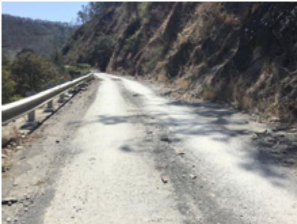
Plate 6.1 Kempsey Road - Lower Creek - Narrow Access
