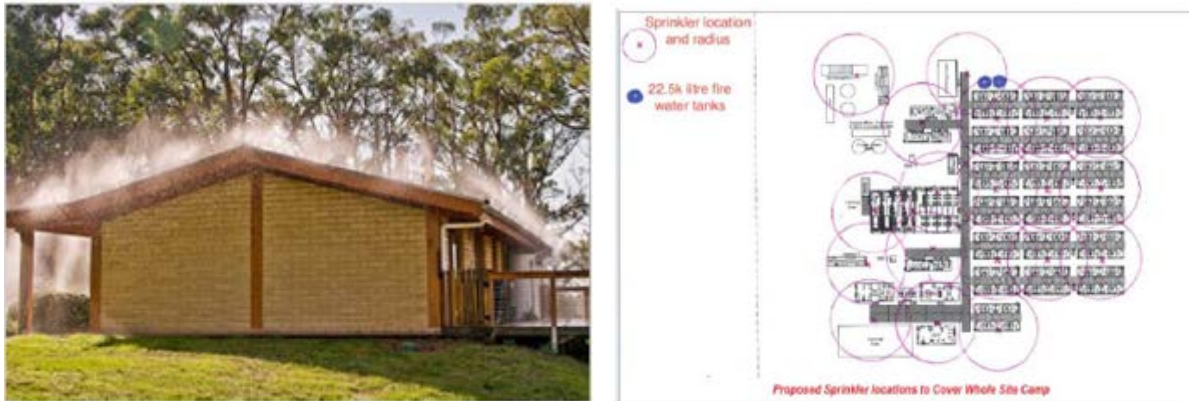
Figure 4.1 Bushfire Sprinkler System
