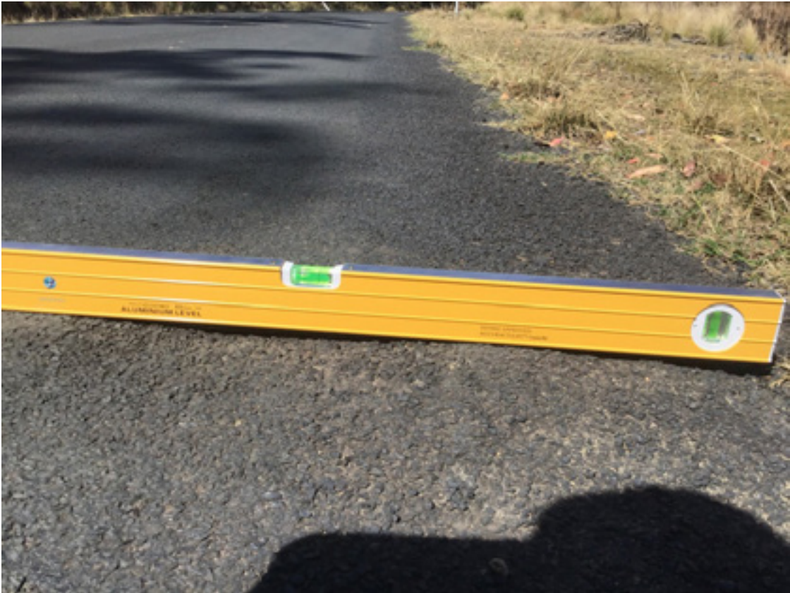
Plate 4.2 Rutting and depressions observed across seal – South of Styx River Crossing
