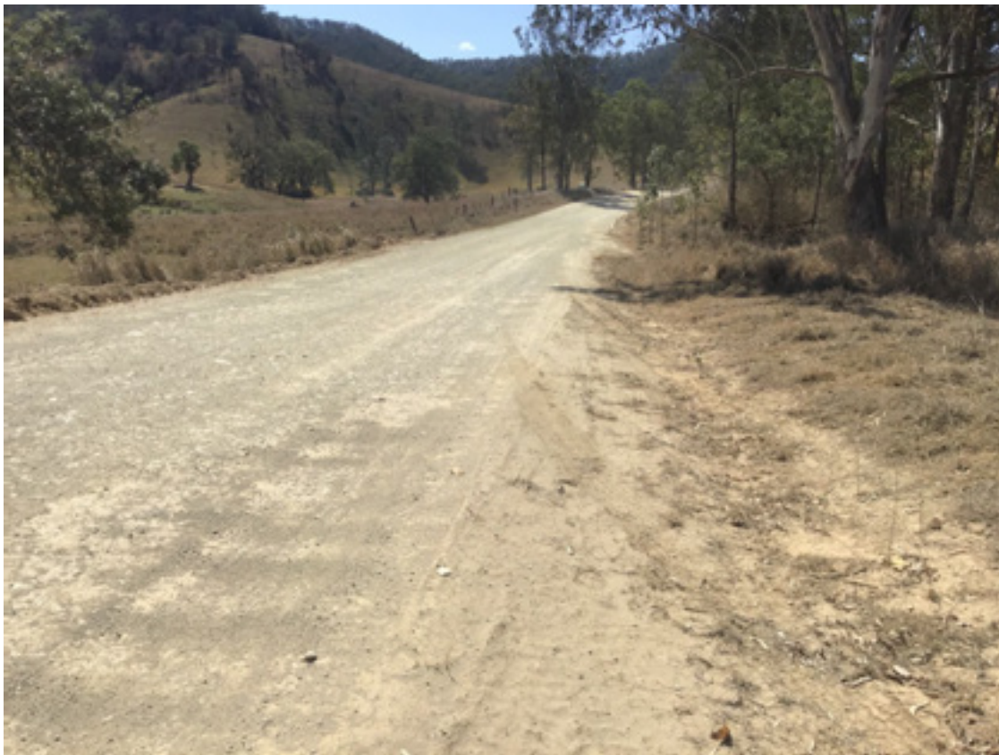
Plate 4.11 Corrugations, protruding aggregates, and loose materials – East of Five Day Creek
