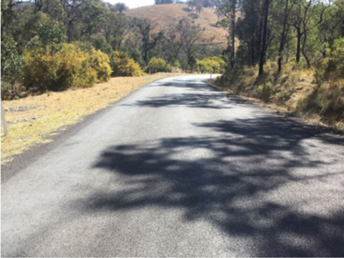
Plate 4.1 Good Condition Sealed Surface – South of Styx River Crossing
