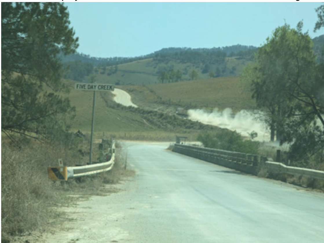
Plate 2.4 Kempsey Armidale Road – Dust Generation on Unsealed Roads
