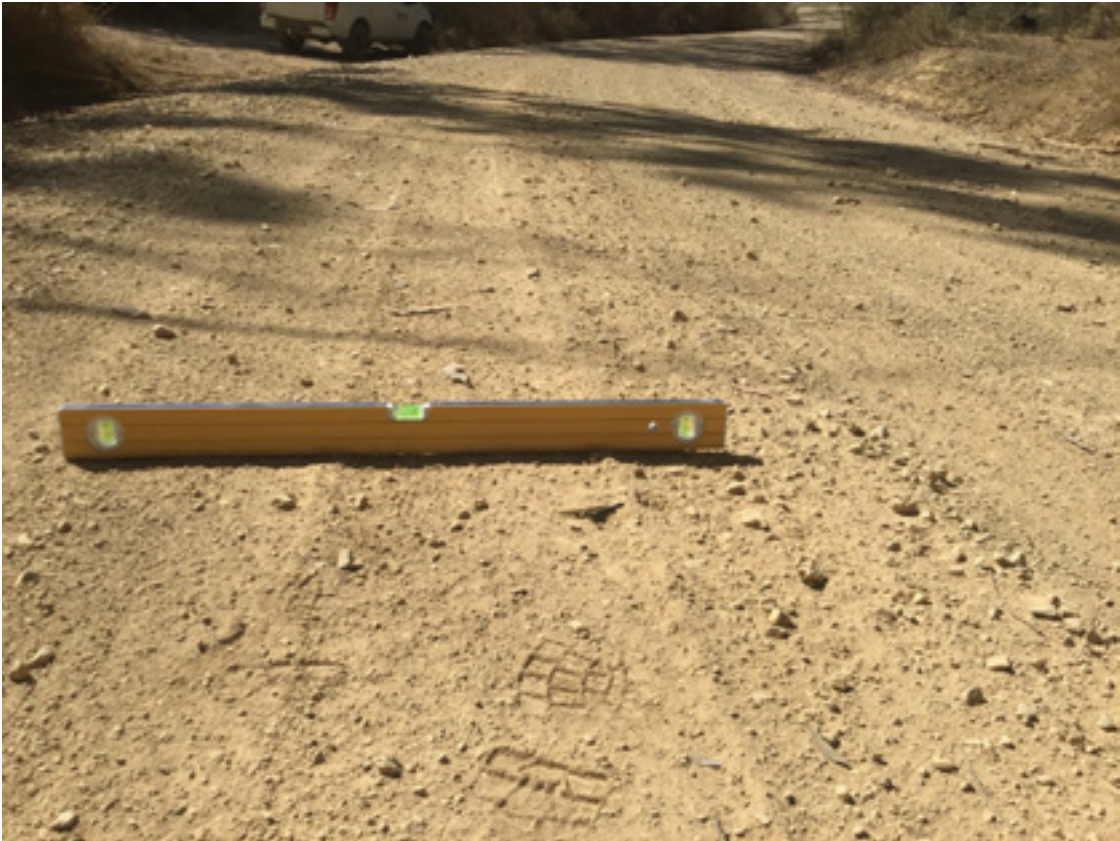
Plate 4.8 Rutting and protruding aggregates/rocks – North of Falls Road
