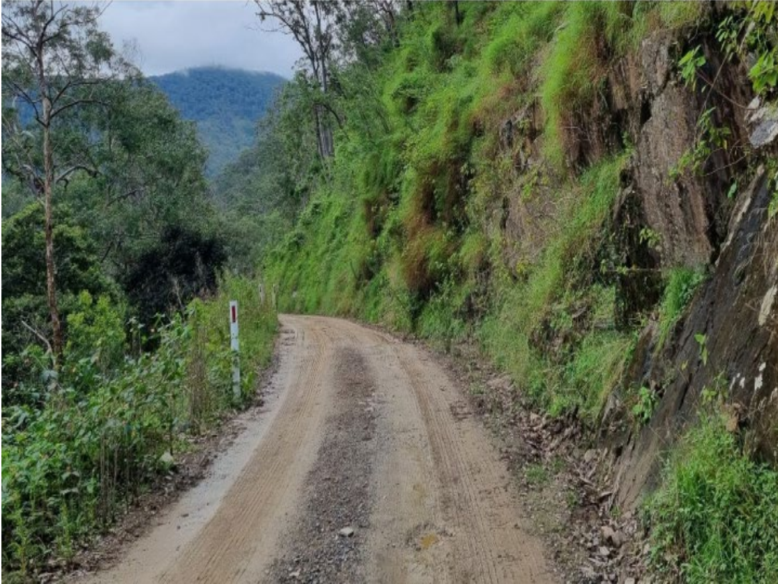
Plate 2.5 Kempsey Armidale Road – Slippery Surfaces During Wet Conditions
