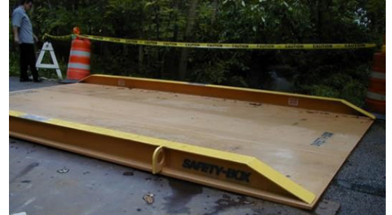
Temporary bridge used to cross open culverts
