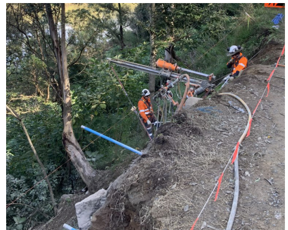
Manual rock drilling with workers suspended in harnesses
