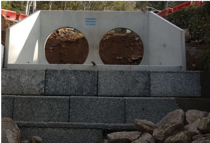
Culvert works at the curves
