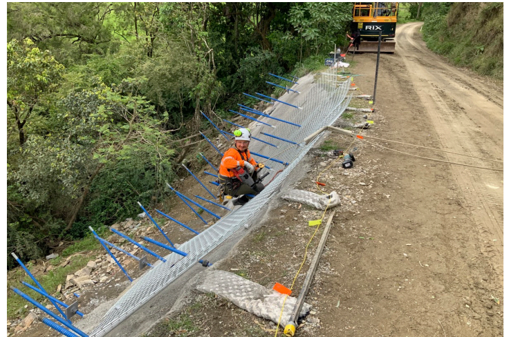
Soil nail wall works at Smith's Bluff
