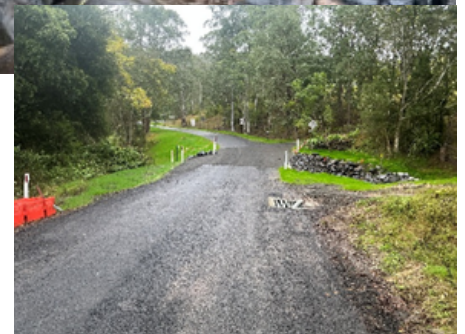
Culvert and remediation work at Flying Fox Cutting
