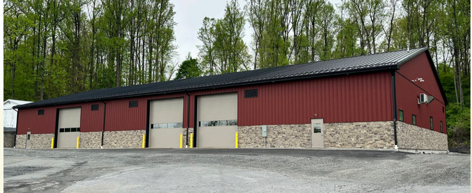
The New Maintenance building was completed in April.
