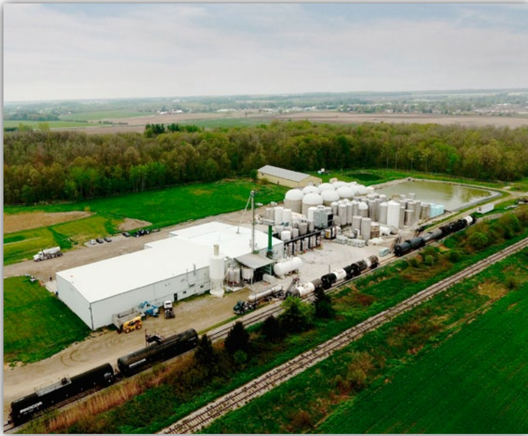
PRODUCTION & DISTRIBUTION NEW HAMBURG, ONTARIO 1356 Nafziger Rd., New Hamburg, ON N3A 3G8
