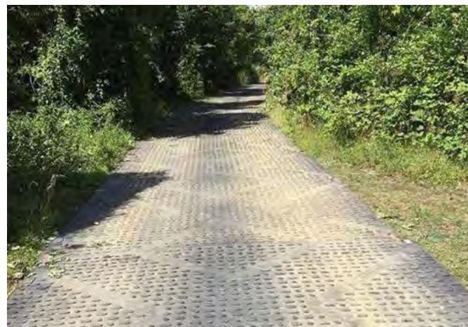
Temporary ground mats
