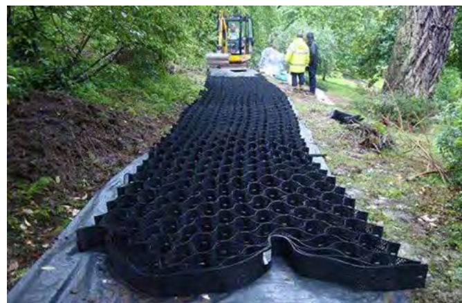
Cellweb ground protection
