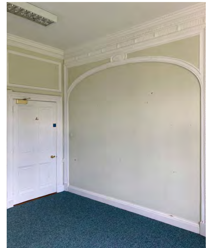
Existing closed-off archway
