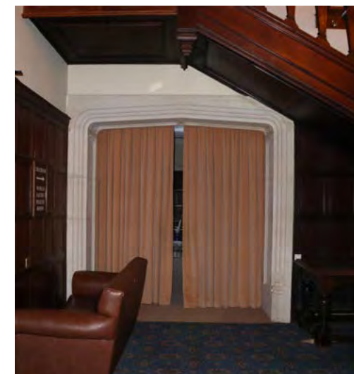
A photograph showing the existing curtain
