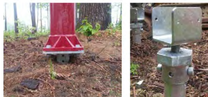
Post anchor connection
