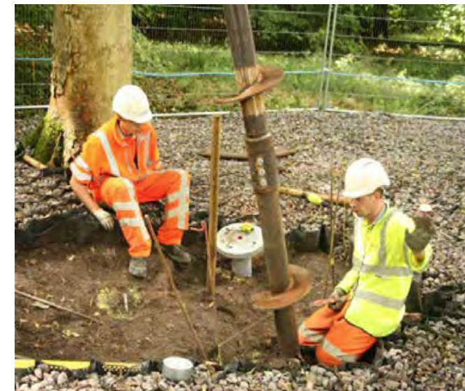
Screw pile installation
