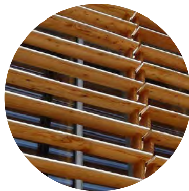
Timber horizontal louvers
