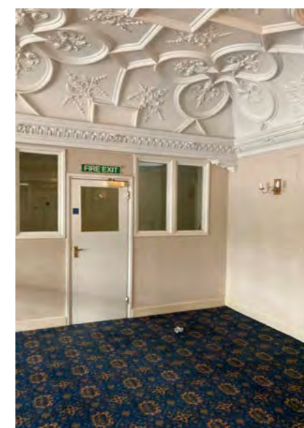
The existing second floor partitions to be retained
