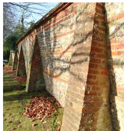
Existing brick boundary walls at Amport House
