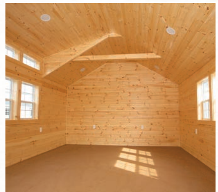
1" x 6" pine finish, recessed lights, pine trim windows, pine baseboard & ceiling trim
