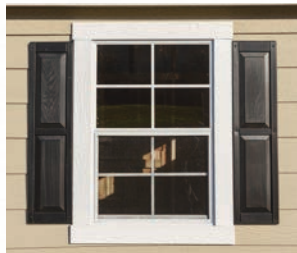
Window Trim & Raised Panel Shutters
