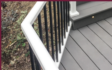
Special Welded Corners
