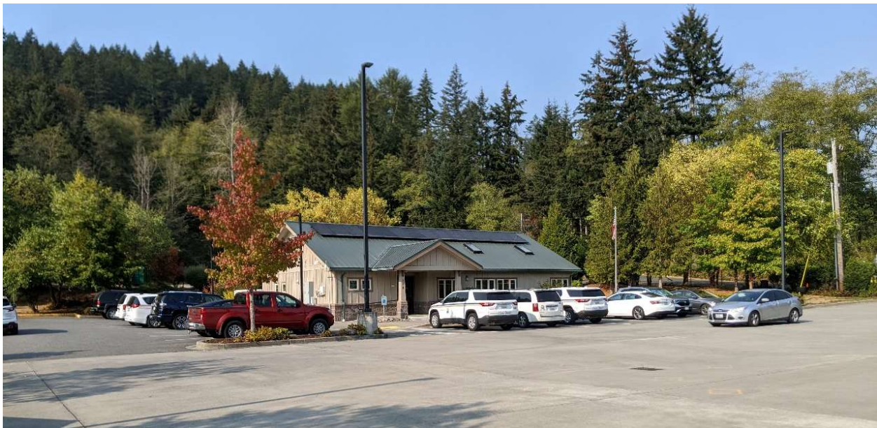
Figure 5 Camano Island Facility
