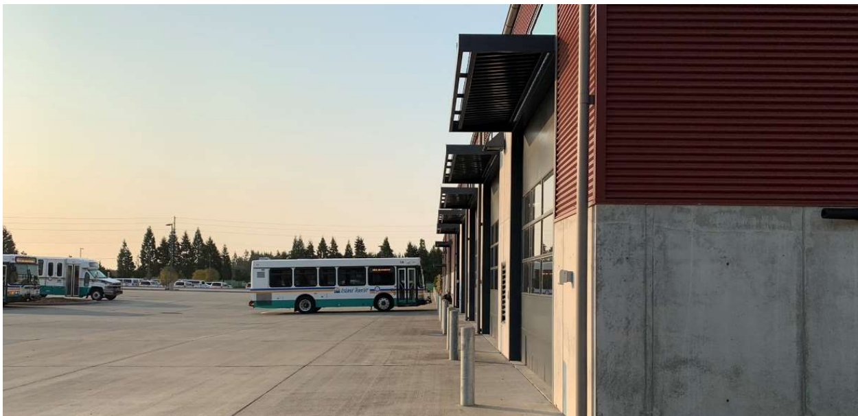
Figure 3 Whidbey Island Facility Maintenance Building and Outdoor Vehicle Storage
