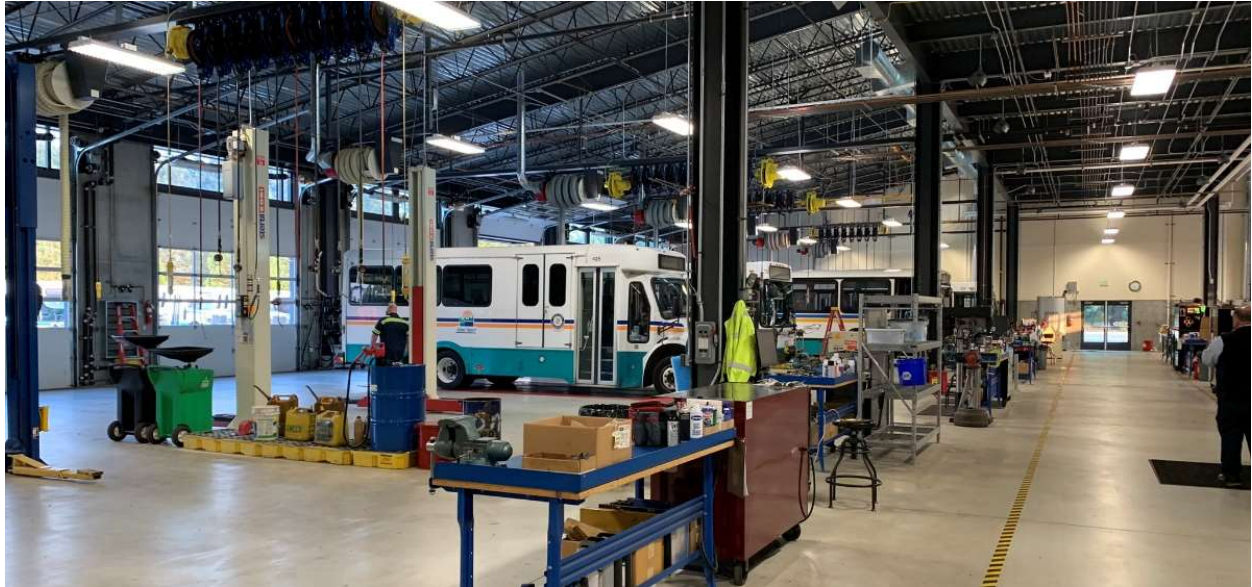
Figure 4 Whidbey Island Facility Maintenance Building Interior
