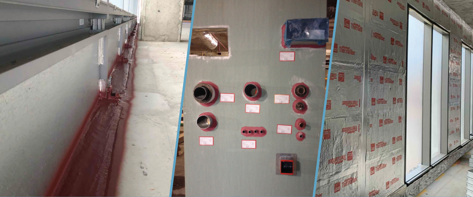
Slab Edge Installed
